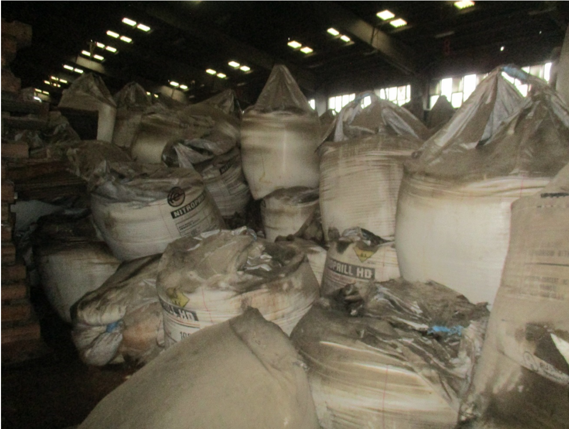
Photograph of the ammonium nitrate bags stored haphazardly on top of each other in hangar 12 in Beirut's port, with some bags looking partly empty, taken in 2020. © 2020 Private
