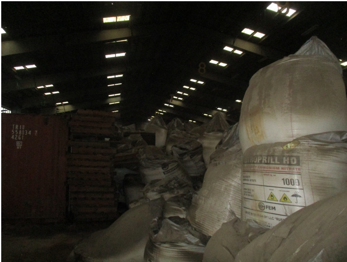
A photograph taken in 2020 of the ammonium nitrate bags stored haphazardly in hangar 12 in Beirut's port. © 2020 Private
